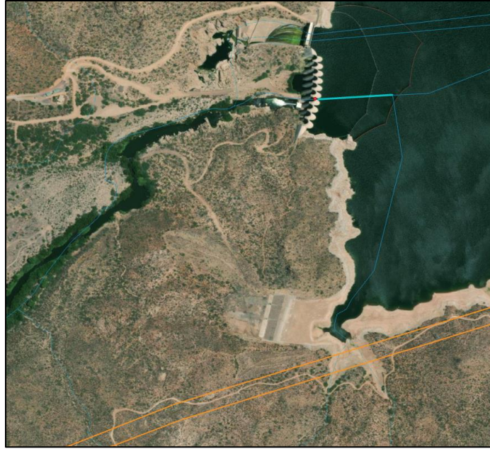
Figure 3: Zoomed in aerial view of Bartlett Dam, where we see it's buttress-type structure, and the highlighted blue line that gave us details on an annual mean flow of 692 cfs.
